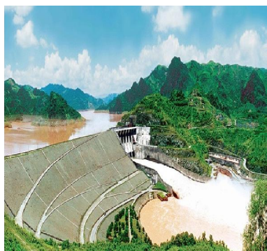
(b) Hoa Binh Dam and Hydroelectricity Plant
